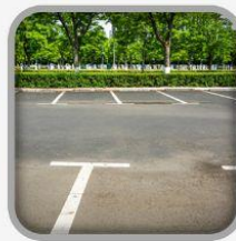
Asphalt Parking Lot
